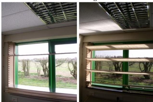
Fig. 4 Louvres in light-shelf (left) and sunshade (right) modes [15]
