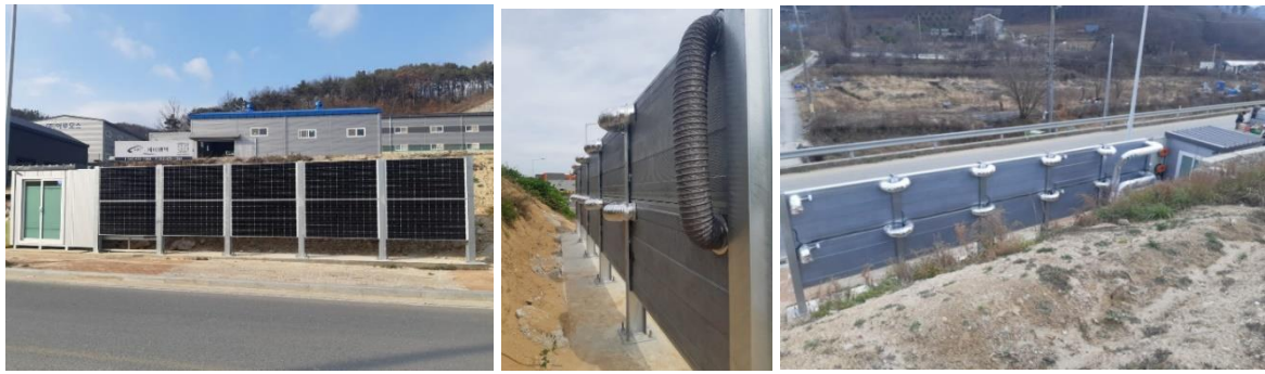
Fig.19. Picture of PV thermal Noise barrier details
