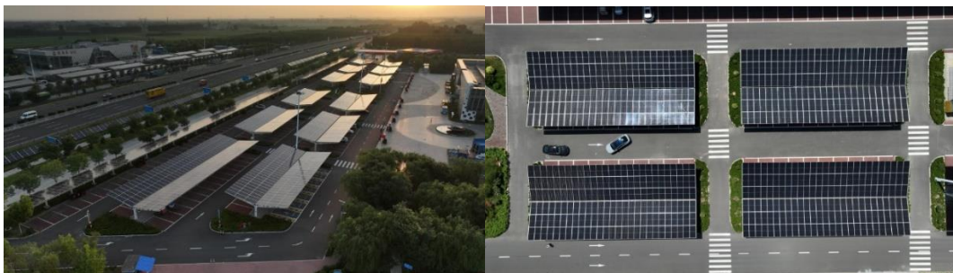
Fig .18. PV Canopy of Jinan East Service Area
