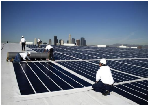
Fig.5. PV membrane installation on the roof directly without mounting system
