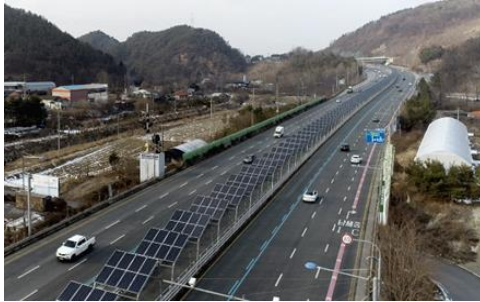
Fig 8. PV mounted in spare Ground
