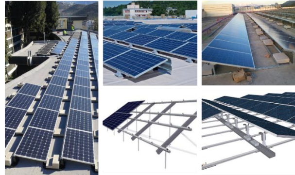
Fig.6. examples of Ballasted mounting systems
