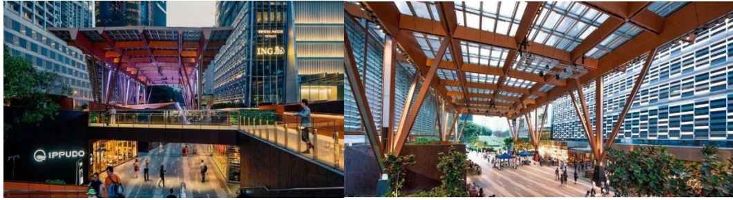
Fig.16. Picture of PV Canopy in Tanjong Pagar Building
