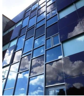
Fig.17. Poly solar opaque series panels (4.6 kWp), Future Business Centre, Cambridge. [20]
